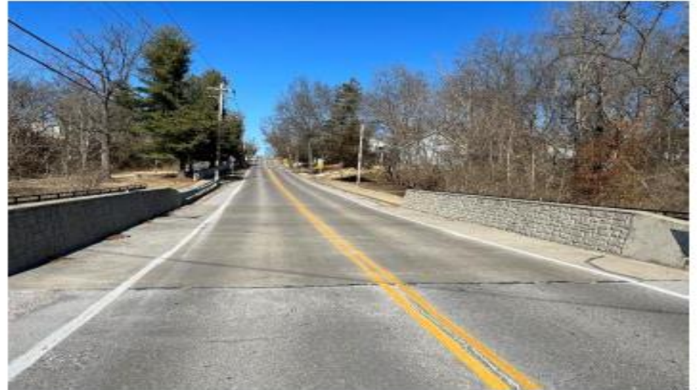
Bridge exception for paving along Hanna Road
