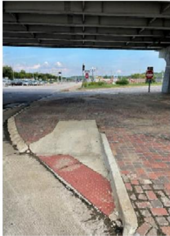
Curb ramps and sidewalks will be replaced under Hwy 141. Pedestrian signal heads and high-visibility crosswalks will be added.
