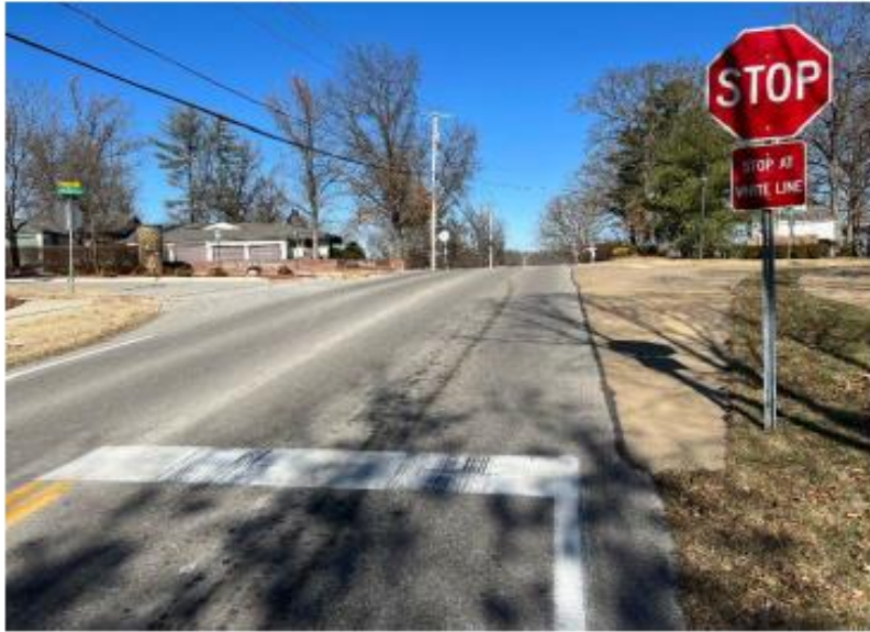
LED Stop signs and high visibility crosswalks will be added at along Hanna Road at the Delmonico Dr intersection
