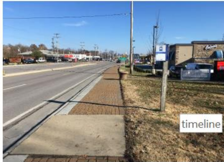
The existing bus stop along Metro Route 57 (Stop ID# 5185) will be upgrade including a new ADA compliant loading/unloading pad, a bus shelter, and bench. The remaining 4 bus stops, within the project limits, will receive upgraded ADA concrete landing pads and benches (where suitable),
