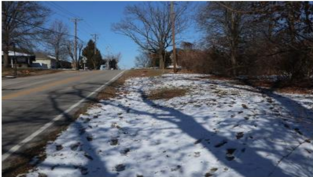
New 5' sidewalks will be added to areas within the corridor without sidewalks
