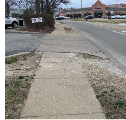
Sidewalk Cracks
