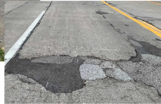
Severe Joint and Crack Spalling, Poor Patching
