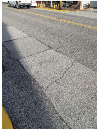
Parking lane Cracking
