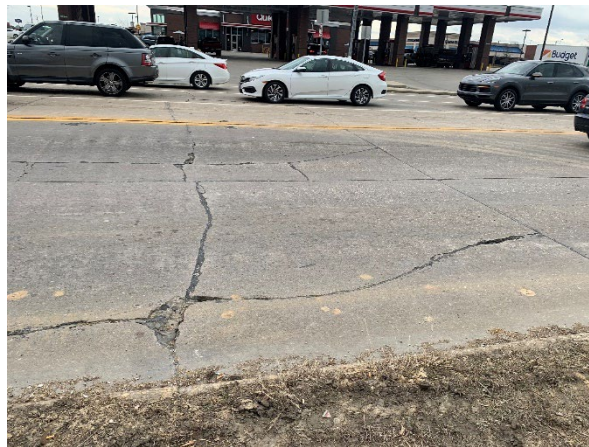
Extensive Cracking
