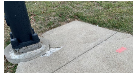
Cracked/Faulted Sidewalk
