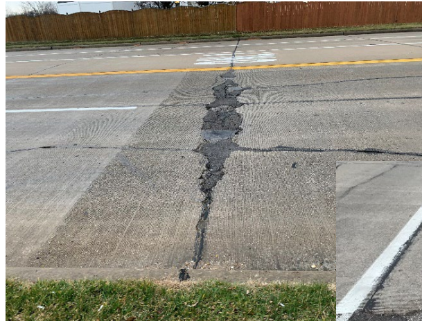
Severe Joint and Crack Spalling, Poor Patching
