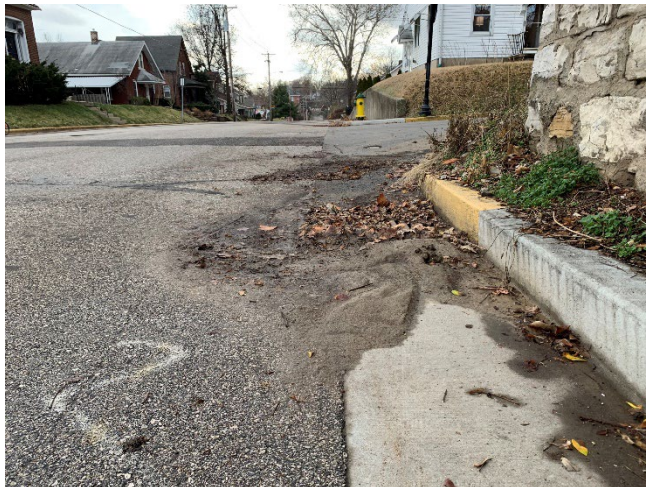
Poor Drainage
