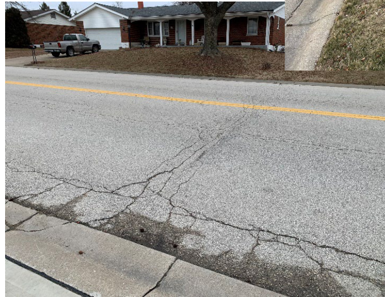
Severe cracking
