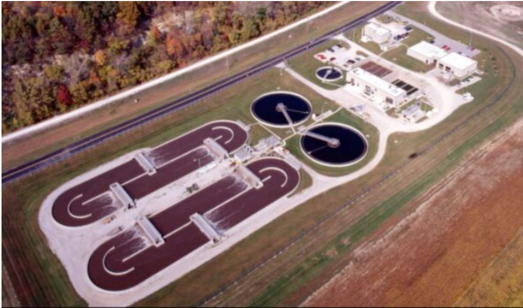
Treatment Plant #1 on Green's Bottom Road at the end of Jung's Station Road.
