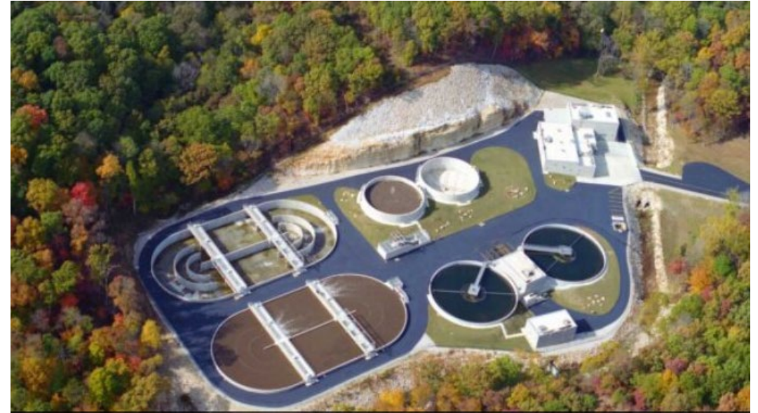
Treatment Plant #2 in the Missouri Research Park near the intersection of Highway 94 & Highway 40/61.
