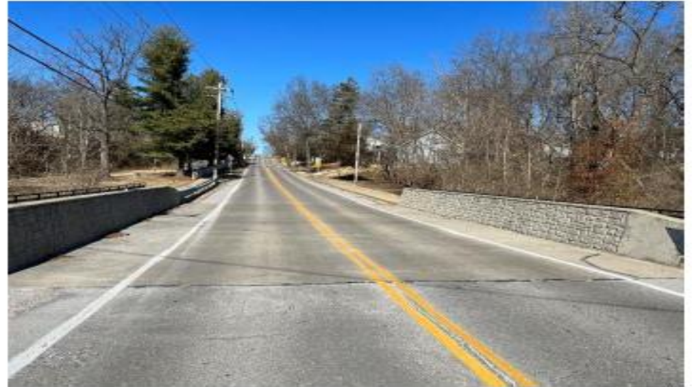
Bridge exception for paving along Hanna Road
