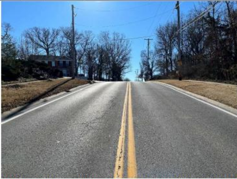
Existing Hanna Road pavement (to be milled and overlaid with an 2" Asphalt Surface)
