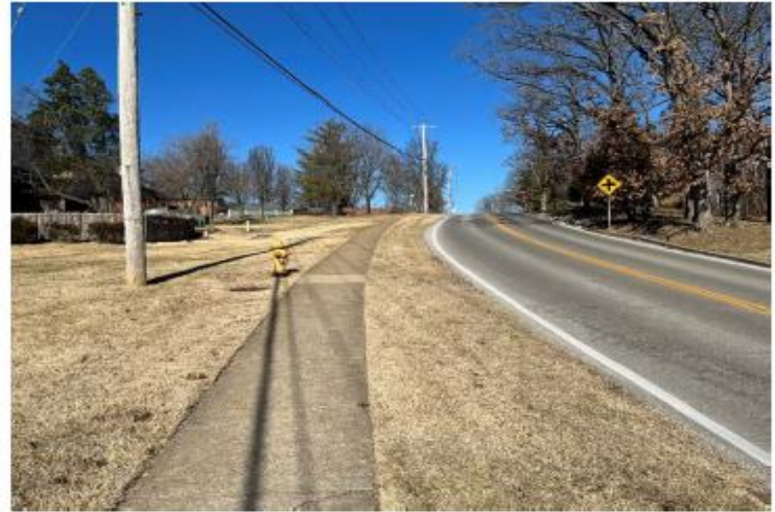
Existing 4' sidewalks will be replaced with new 5' sidewalks (both sides of the road)
