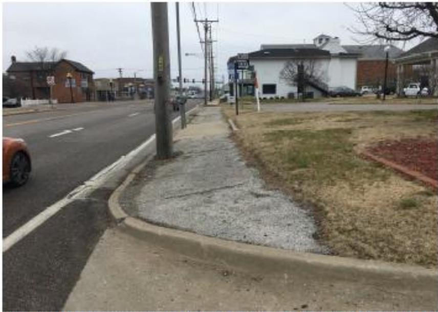
A few short, but non-contiguous sections of sidewalk/asphalt shoulder, do exist along the north side of Manchester Road. These sections are non-ADA compliant and collectively do not establish a sidewalk system.
