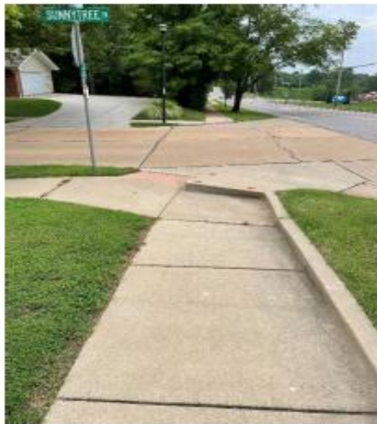
Non-ADA complaint curb ramps (on the south side of Carman) will be replaced
