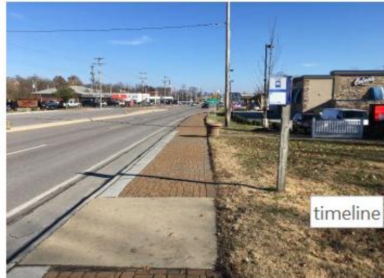
The existing bus stop along Metro Route 57 (Stop ID# 5185) will be upgrade including a new ADA compliant loading/unloading pad, a bus shelter, and bench. The remaining 4 bus stops, within the project limits, will receive upgraded ADA concrete landing pads and benches (where suitable),
