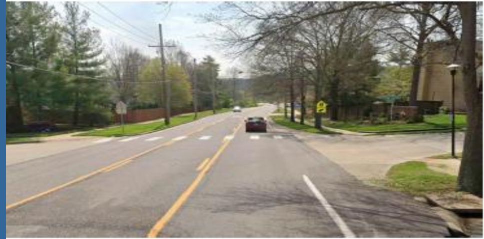
Carman Road and Stone Canyon mid-block crossing solar powered Rectangular Rapid Flashing Beacon and high visibility continental crosswalk will be installed.
