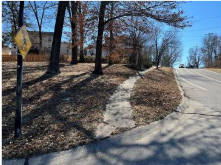
Curb ramps will added (where they do not currently exist). Non-complaint curb ramps will be replaced
