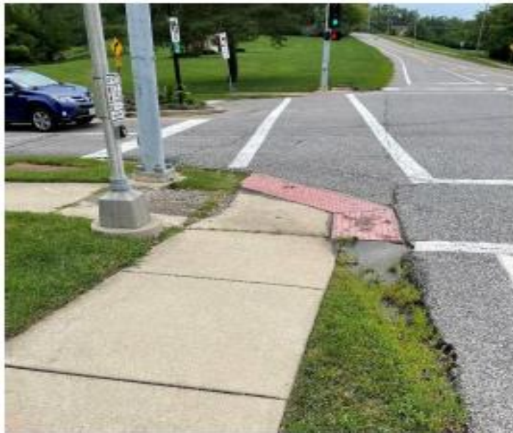
Beginning of project – south side of Carman Road
