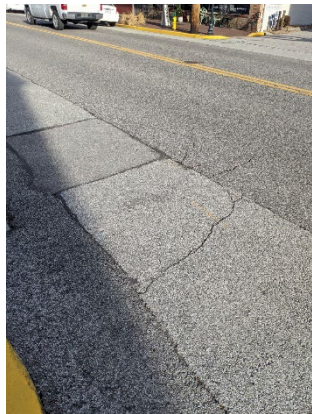
Parking lane Cracking
