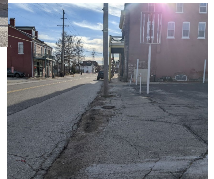
Inadequate Sidewalks and Curb Ramps
