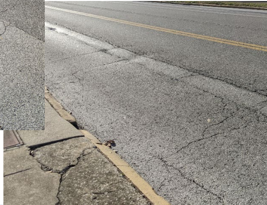
Parking lane Cracking
