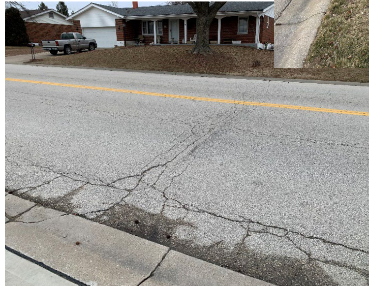
Severe cracking
