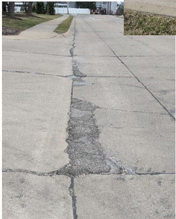
Severe Joint Spalling
