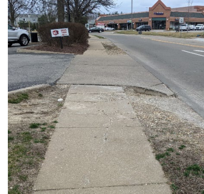
Sidewalk Cracks
