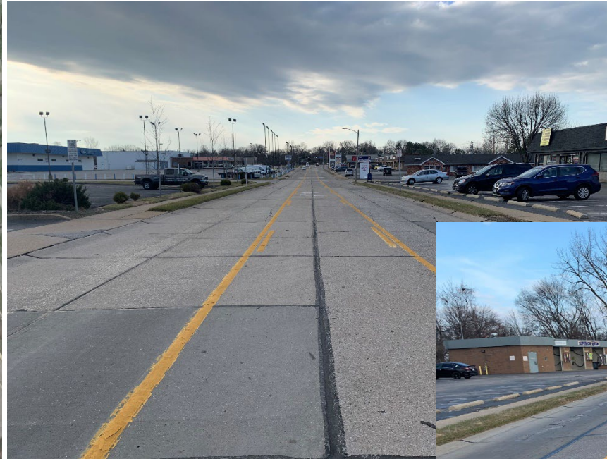
Duchesne Drive at old Pundmann Ford looking south towards West Clay Street
