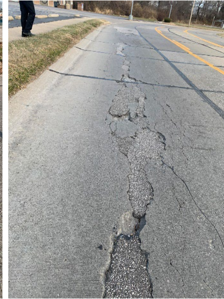
Extensive Cracking
