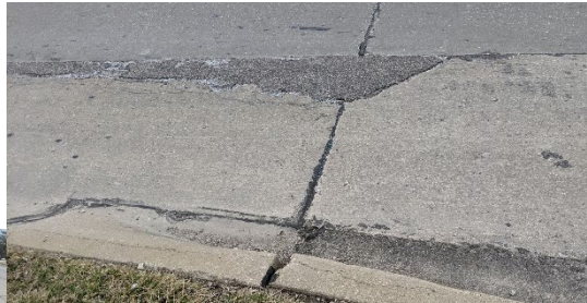
Severe Joint Spalling
