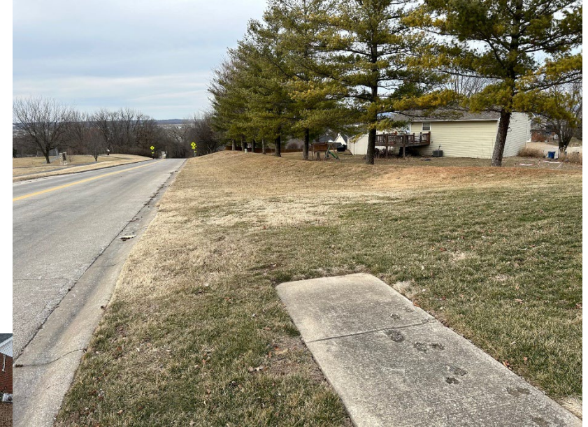
Sections of missing sidewalk
