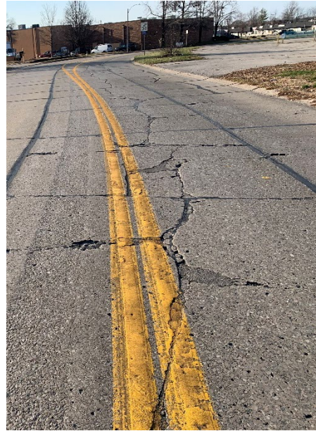
Extensive Cracking
