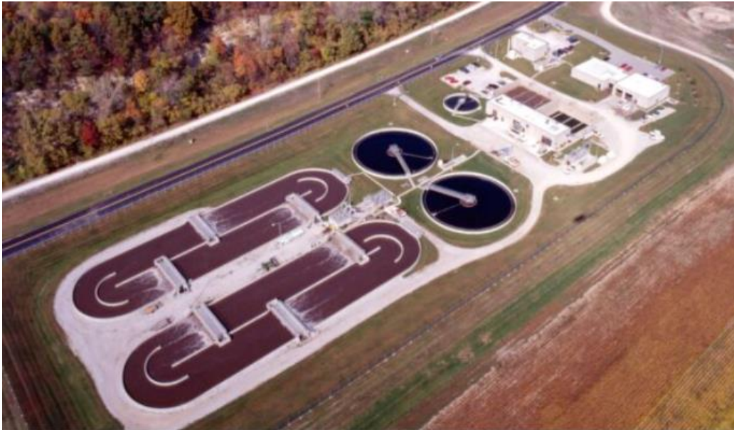
Treatment Plant #1 on Green's Bottom Road at the end of Jung's Station Road.
